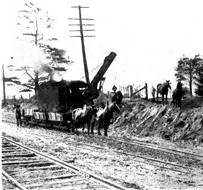
Fig. 3—West of the Etobicoke Creek, a maximum grade of 6 per cent. has been reduced to 1 per cent.
